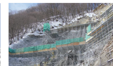
Can be erected along slopes and also used as a gantry YT Lock System
